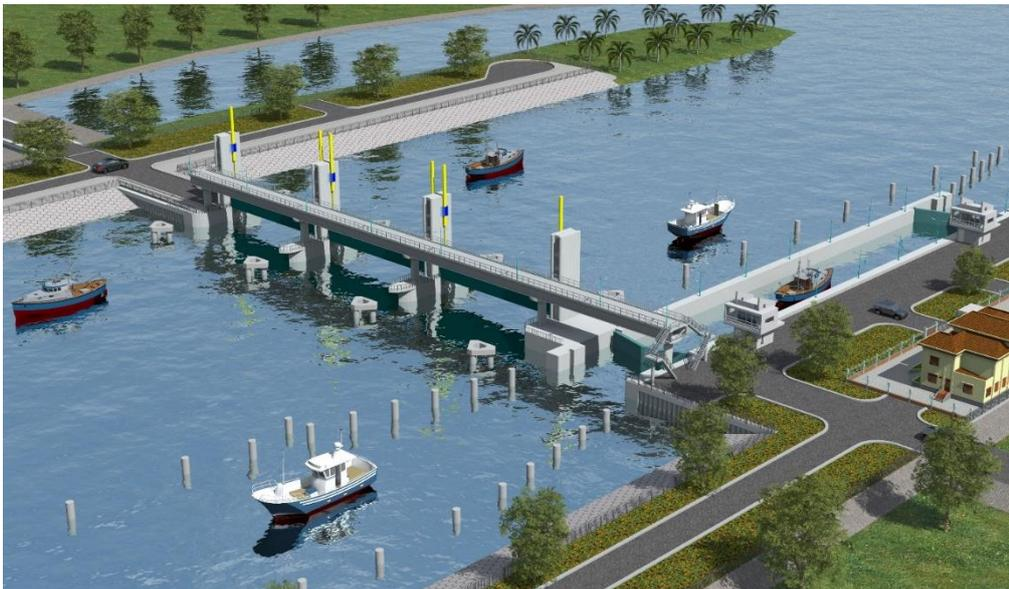
Photo: Example of one of the flood barriers, design based on Dutch 'Hartelkering' (with courtesy of TrungNam)
